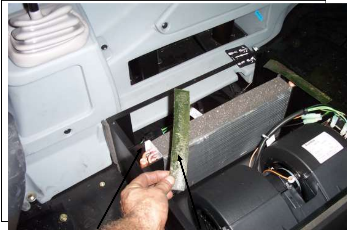
Tar paper gasket was here( same on other end of coil)
