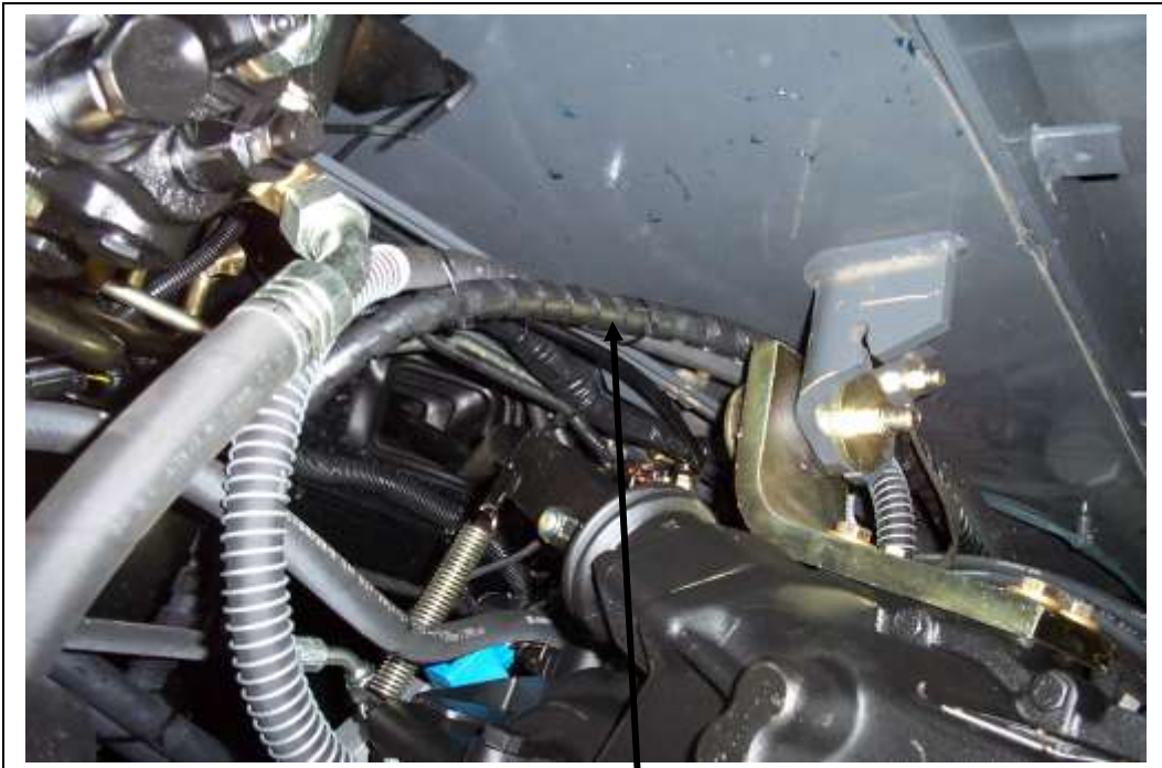
5/16" hose running along the right main frame rail from the drier back towards the rear axle
