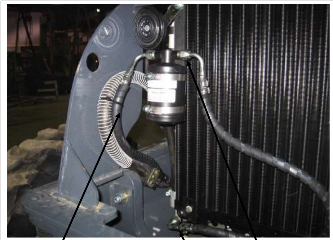
5/16" 90° fitting at drier outlet on long 5.16" hose.
