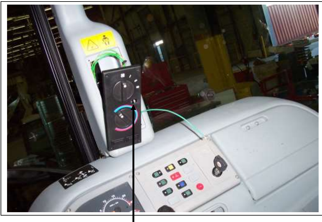
5/8" hole drilled for AC on/off pushbutton switch
