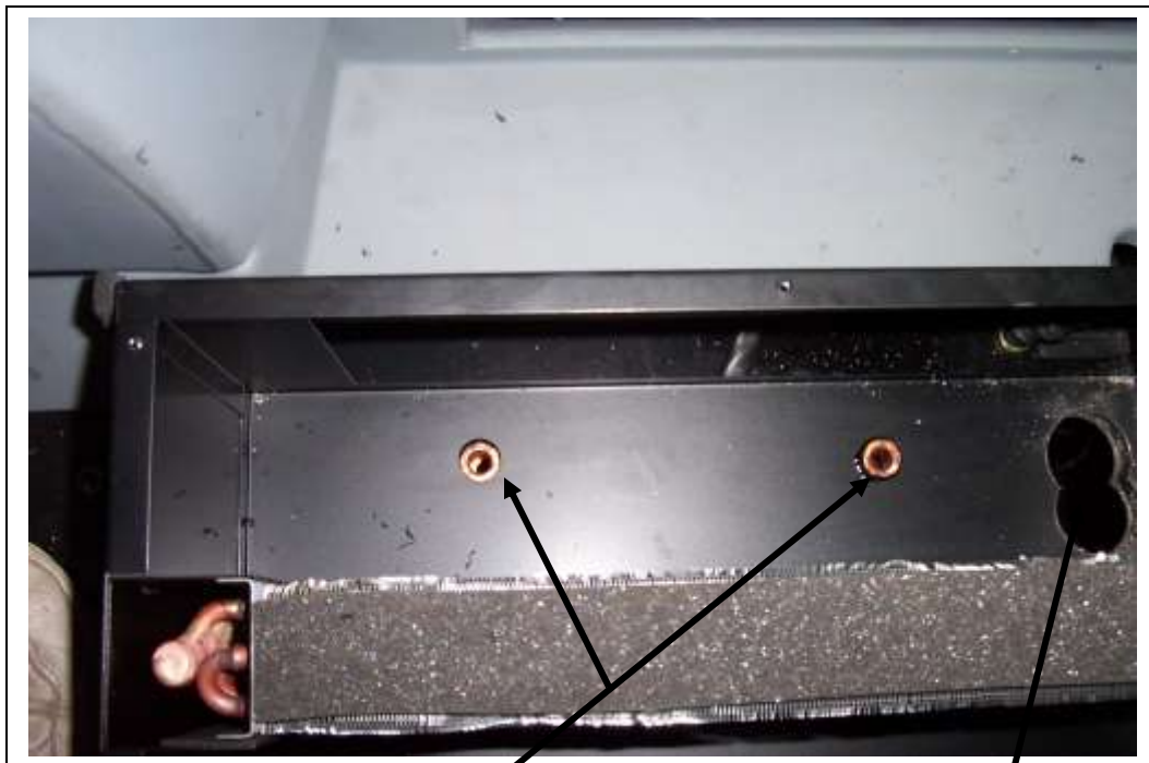
Copper glue in drain tubes. Drill a 1/2" hole through both layers of the box floor . Glue in using epoxy
